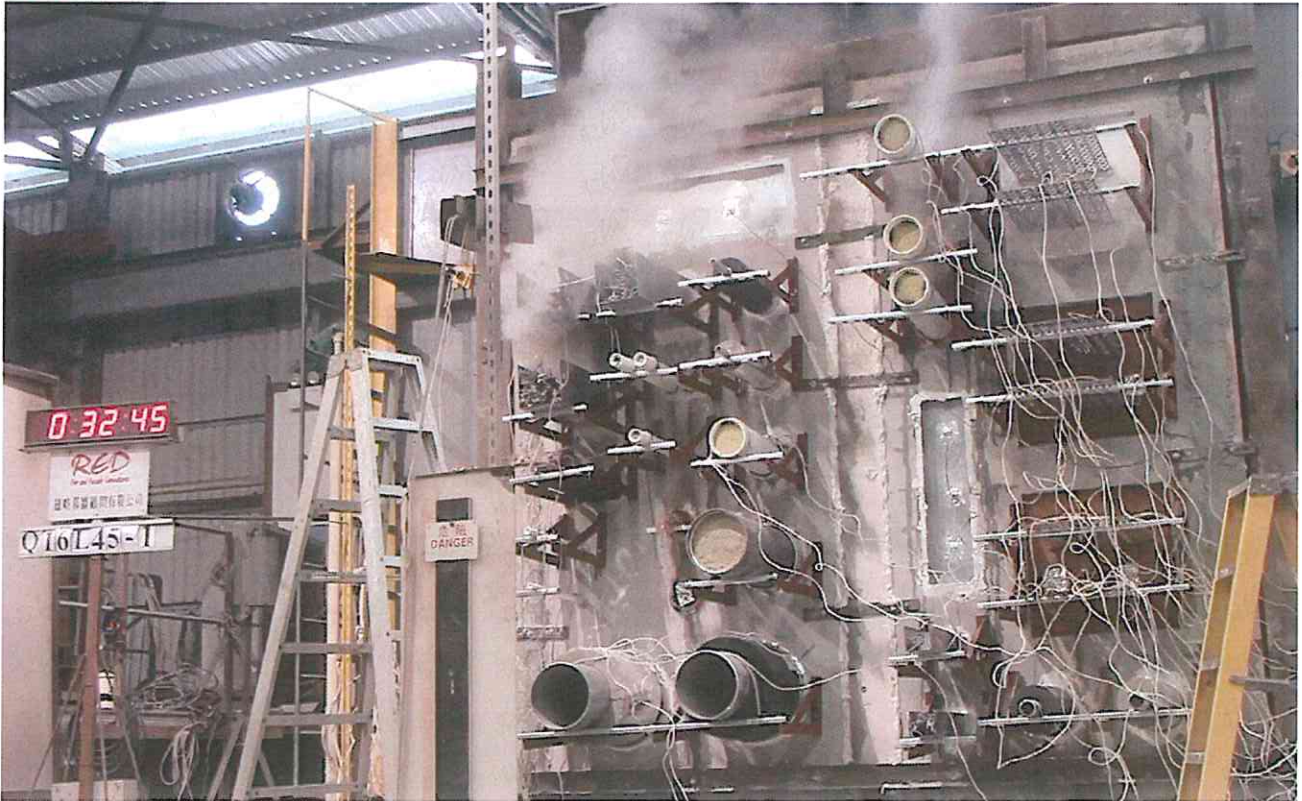
Photo 2: The unexposed face of the specimens after a heating period of 32 minutes.
