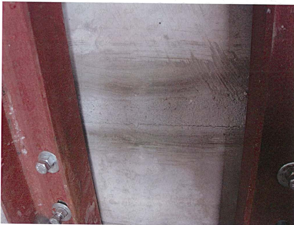
Photo 3: Specimen A after the test, the upper interface detached from the concrete substrate
