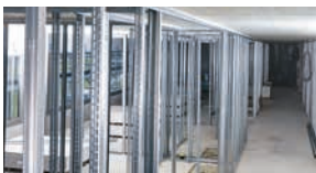
Drywall tracks to concrete and steel
