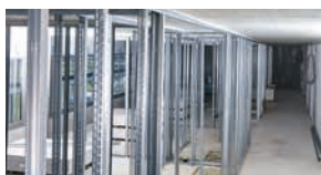
Drywall tracks to concrete and steel
