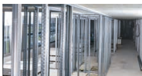
Drywall tracks to concrete and steel
