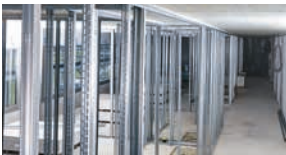
Drywall tracks to concrete and steel
