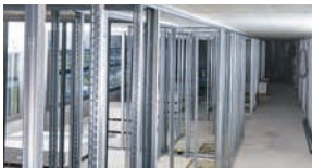
Drywall tracks to concrete and steel
