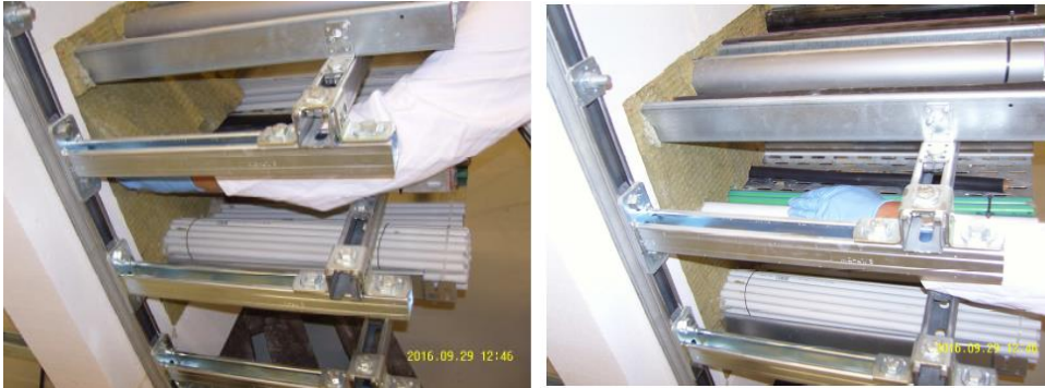
Fig. 6: Cutting and fitting mineral wool board [11]
